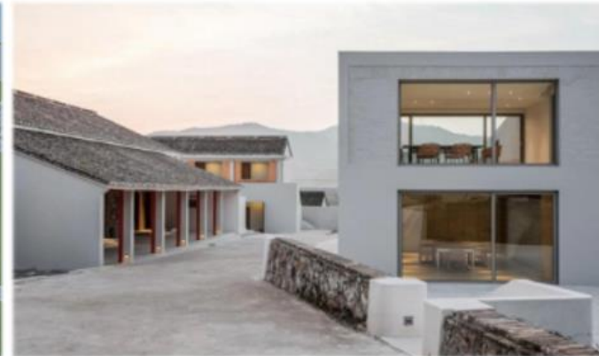
Old House Renovation
