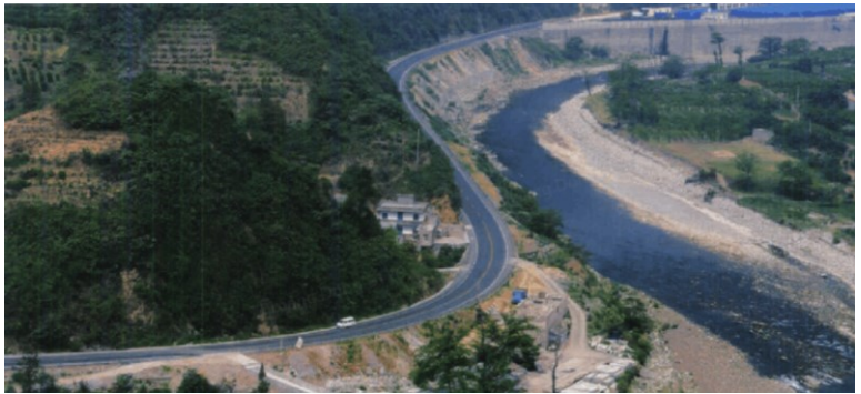
A flat curve consists of straight lines, gentle curves, and arcs.
