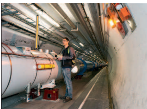
Nedo products in use at CERN
